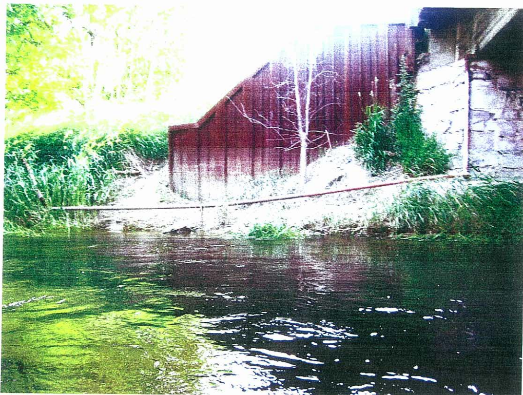
Fig. 3 – Under Chip Road Bridge.
